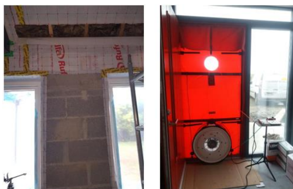
Figure 3: Air Tightness Testing Examples
